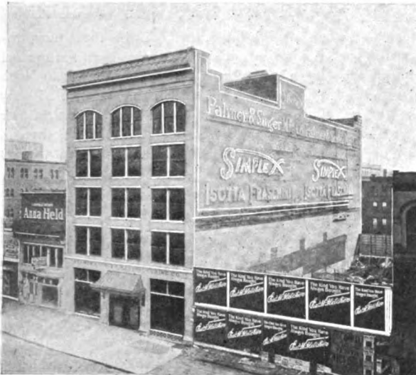
BROADWAY ENTRANCE TO BUILDING.
